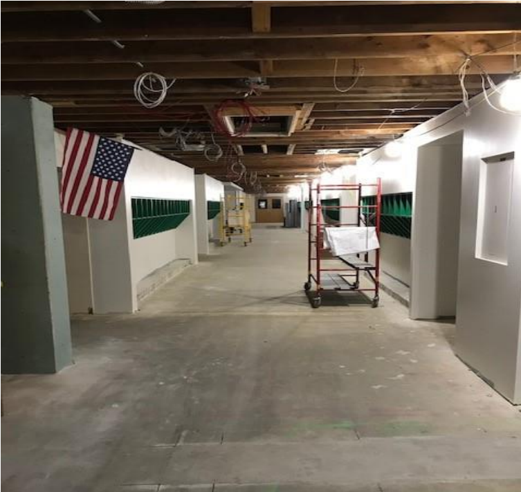
PLE Renovation – Cubbies Installed In 2 nd Grade Corridor
